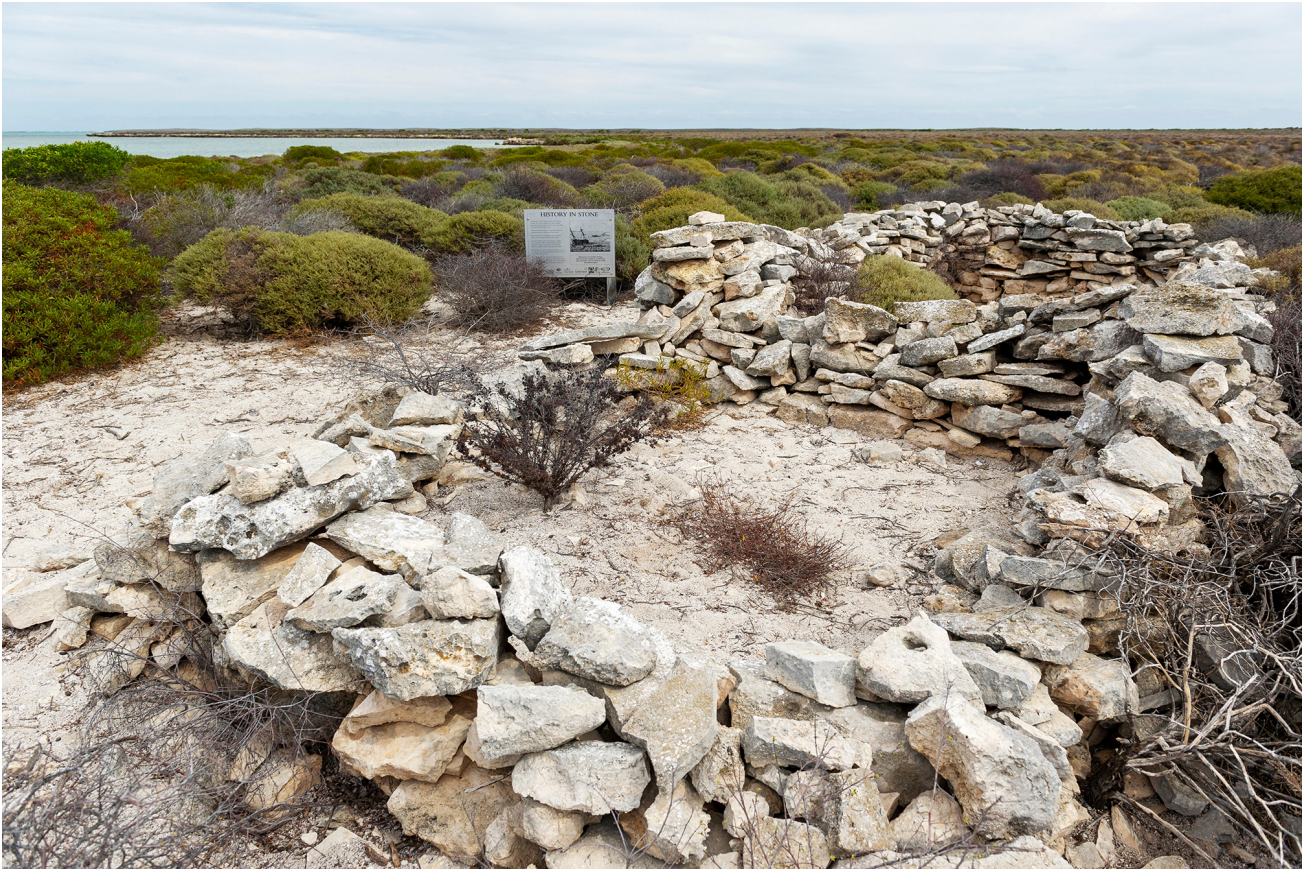
Figure 5. Coastal structure (Wiebbe Hayes Fort) constructed 1629, www.alamy.com image RYPBYW. Note the thin-bedded fine-grained grey limestone (calcrete) forming the building slabs.
